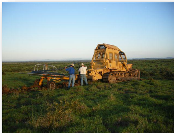
Laying poly pipe for the reticulated water system
