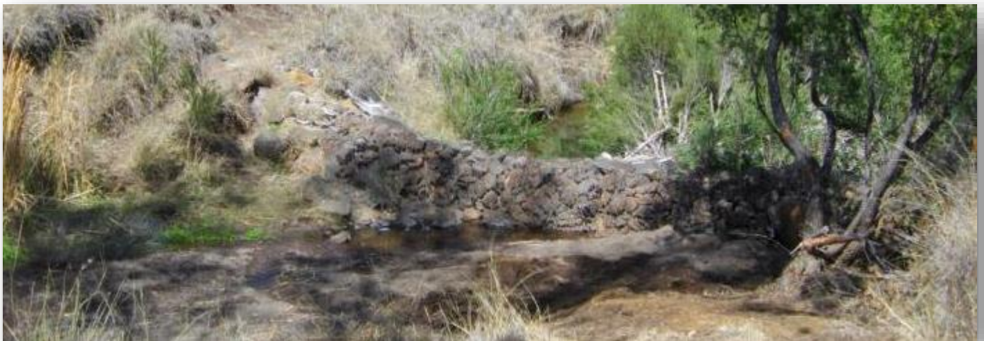
'Leaky weirs' aim to capture and utilise as much water as possible
